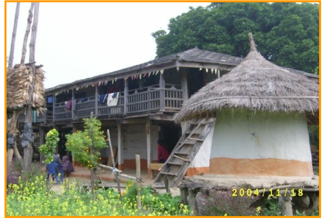
Affected House at Bengadabar VDC
